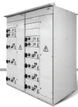
Low Voltage Switchgear & Motor Control Center
