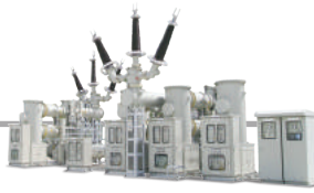
Gas Insulated Switchgear
