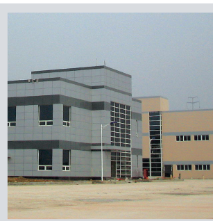
Wuxi Plant (China)
