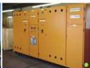
CHINT Products Installed in Switchgears, South Africa
